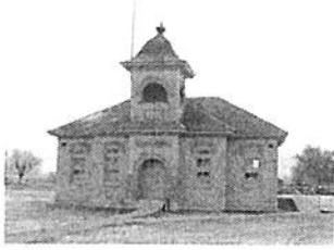
Fairfield School House, 1898
