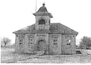
Fairfield School House, 1898
